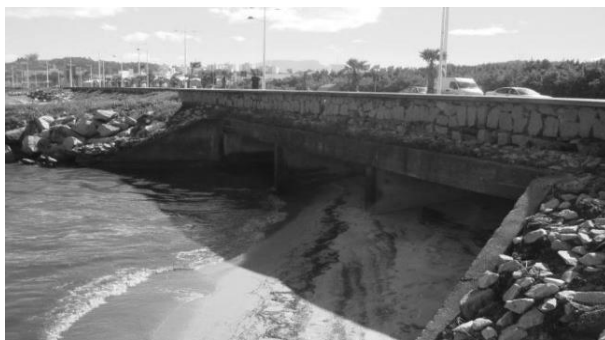
Figure 11. Openings for passage of seawater to mangrove (source: Authors, 2013).
